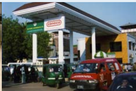
CNG Filling Station
